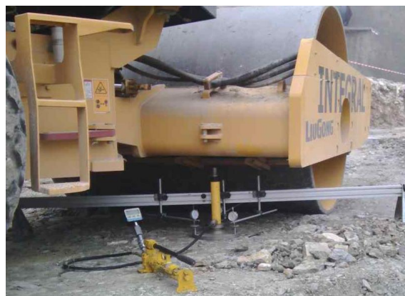
Figure 2. The procedure of measure of static deformability module
