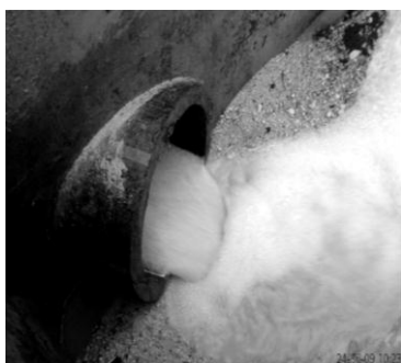
Figure 1. Milk in the drainage system of leachate[5]
