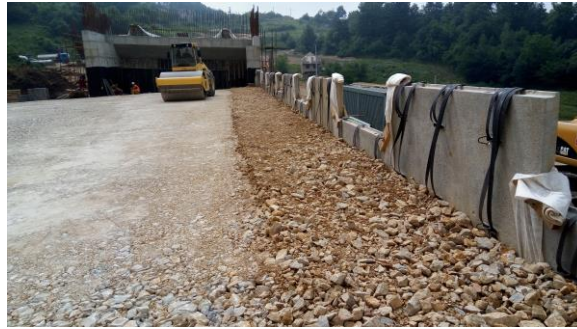
Figure 1. Preparation of layer of reinforced embankment
